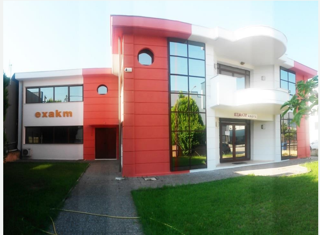
Offices, Labs & Production Plant in Sindos Industrial Zone in Thessaloniki
